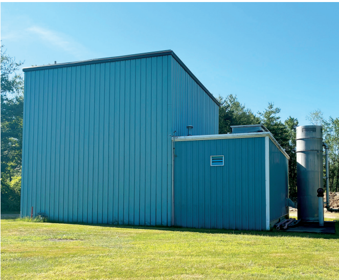
The Clapp/Whitcomb Treatment Plant underwent its last significant modification in 1999. Although it could supply up to 700,000 gallons per day, declining water quality, aging technology, and regulatory changes minimize our ability to rely on this facility.
