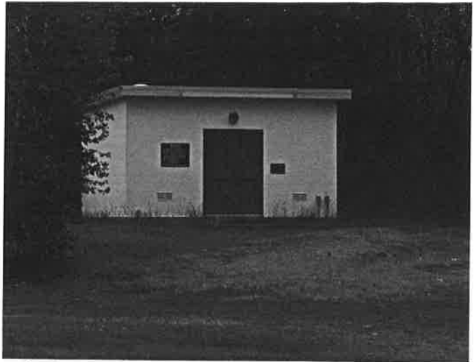
Redevelopment of the Clapp Well in West Acton should make it a more reliable source of drinking water.
