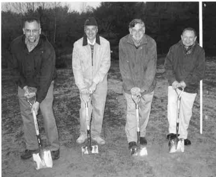
Chris Allen, Acton Water District Manager, and Water Commissioners (from left to right) Ron Parenti, Steve Stuntz, and Len Phillips break ground for the new Kennedy/Marshall Water Treatment Plant.
