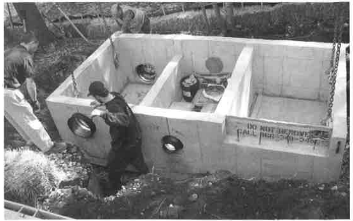
A Filterra basin is installed near the Marshall well on Route 27 in North Acton. The Filterra basin both slows down the runoff of water into the nearby ground and surface water, and filters out many of the pollutants in this runoff.
