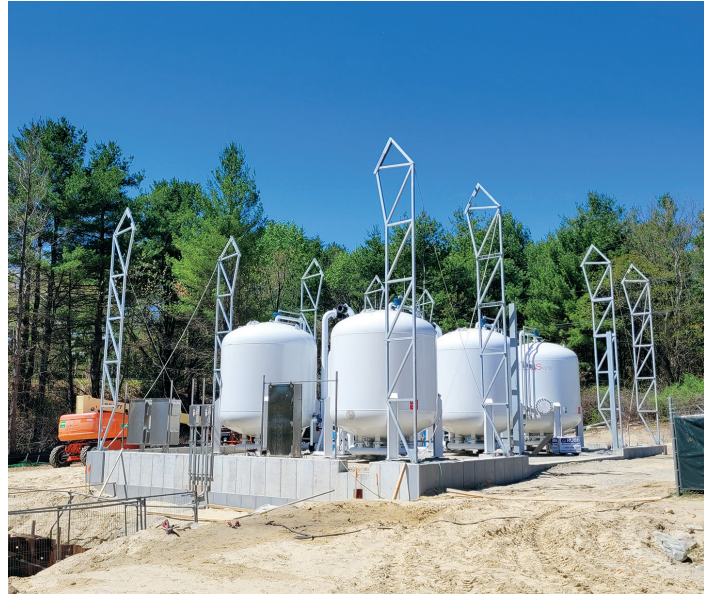
The PFAS filtration equipment was delivered to both South Acton (above) and Center Acton sites in April, we anticipate these systems being operational in the fall of 2025.
